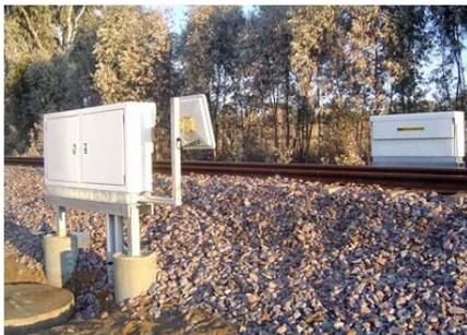
**Figure 6. RailBAM - Bearing Acoustic Monitor [28]**
